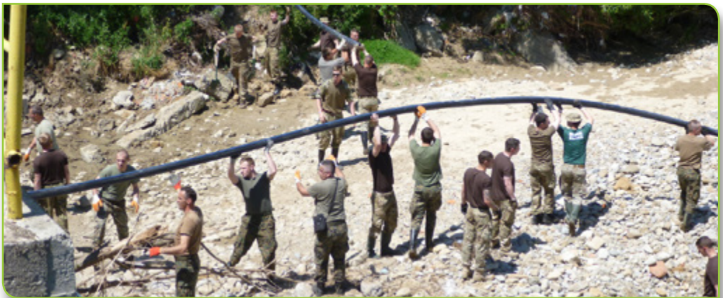
UK and EUFOR soldiers laying pipes in Lopare
