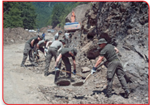
The Austrian Reserve troops deployed for roads reconstruction
